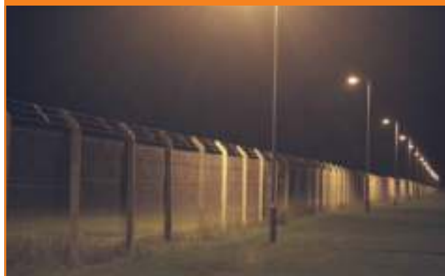
(מקור: Security Lighting – CPNI - Centre for the Protection of National Infrastructure)
