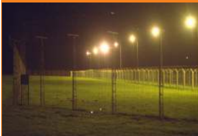
(מקור: Security Lighting – CPNI - Centre for the Protection of National Infrastructure)
